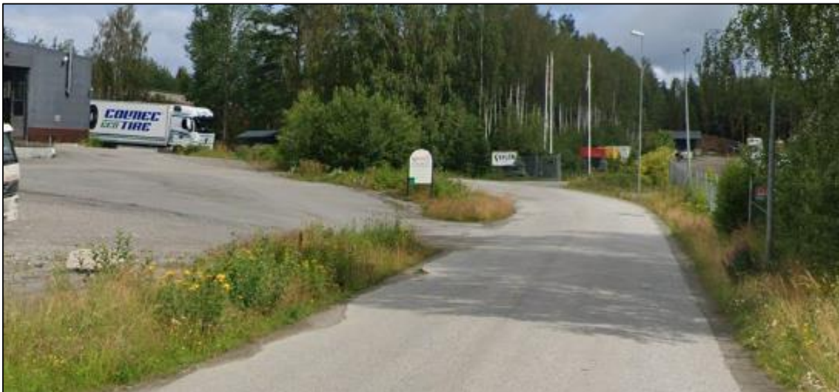
Figur 2.3: Vegen Slomarka (Kilde: Google Streetview)
